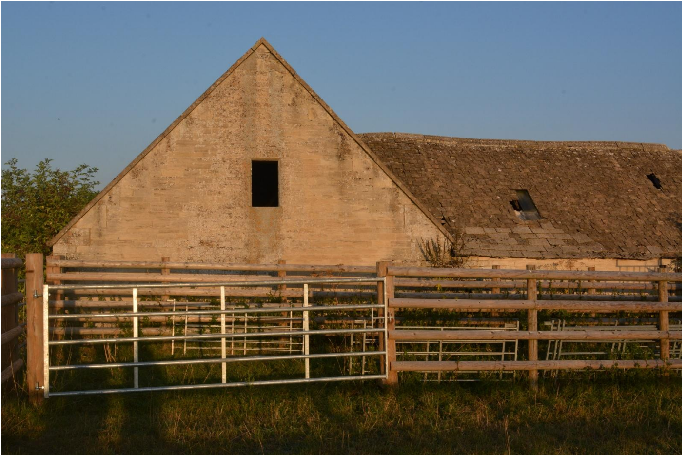
Gable on the western elevation. Note open skylight and concrete replacement slates to the right of the gable.
