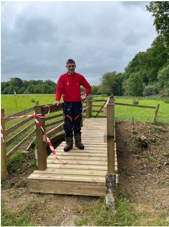
Left : James Bradford, Ranger, and the Bridge replacement at Sabrina Way. Photo Credit. Georgina Lindsay
